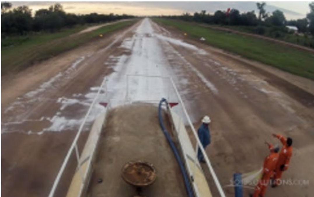
Application of the surface seal
